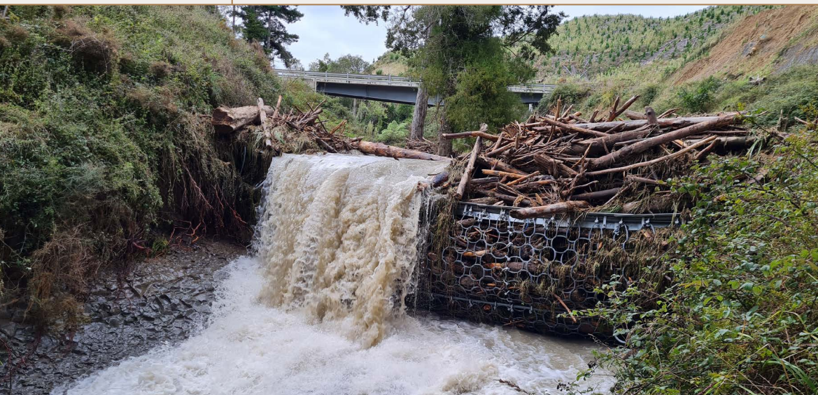
Figure 9. Aerial view of Hampton Forest debris net post weather event
