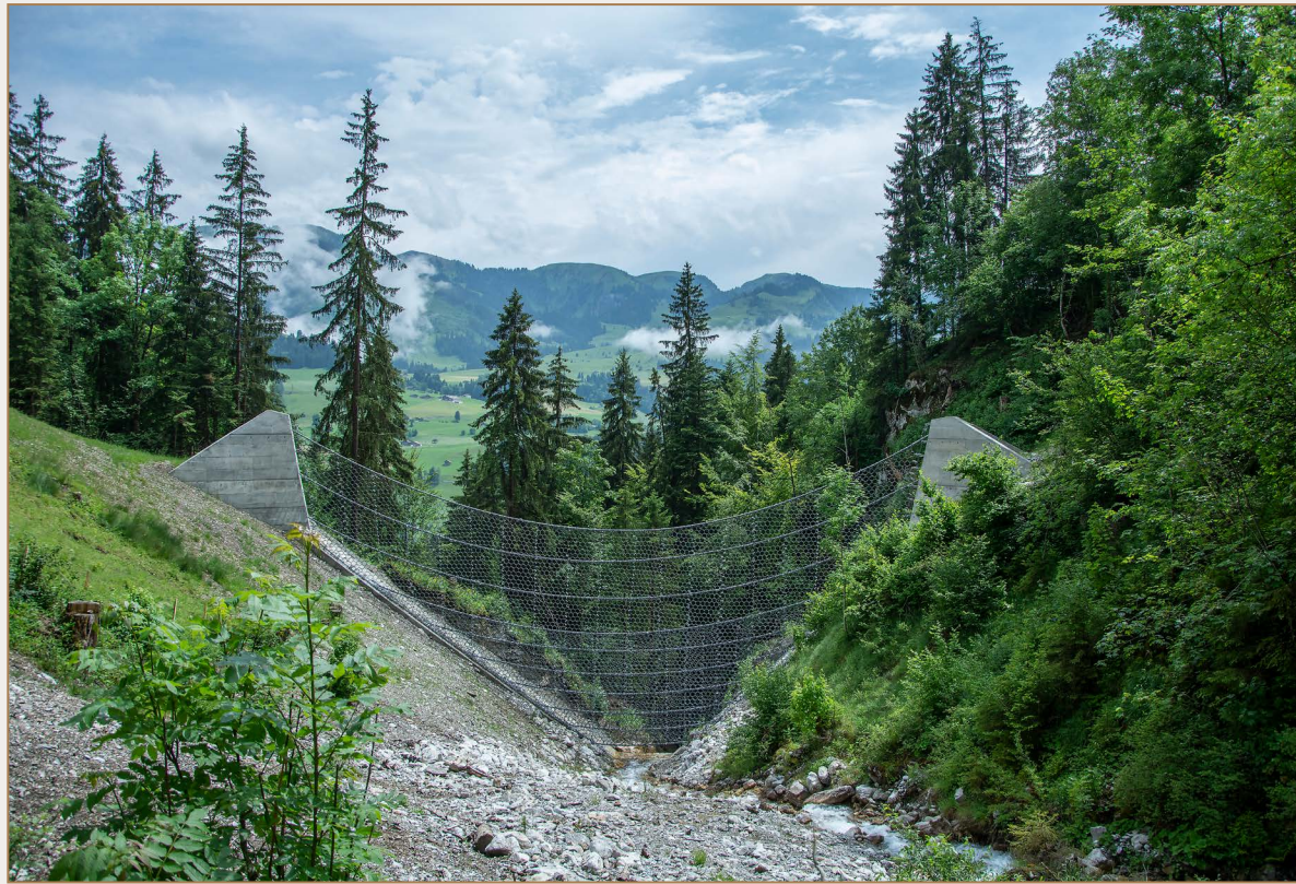
Figure 6. Kaikoura debris nets, installed to protect State Highway 1 and the adjacent railway line after the 2016 Kaikoura earthquake
