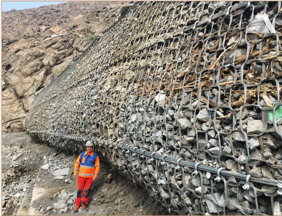
Figure 4. Springs Junction (South Island) – Shallow landslide barrier
