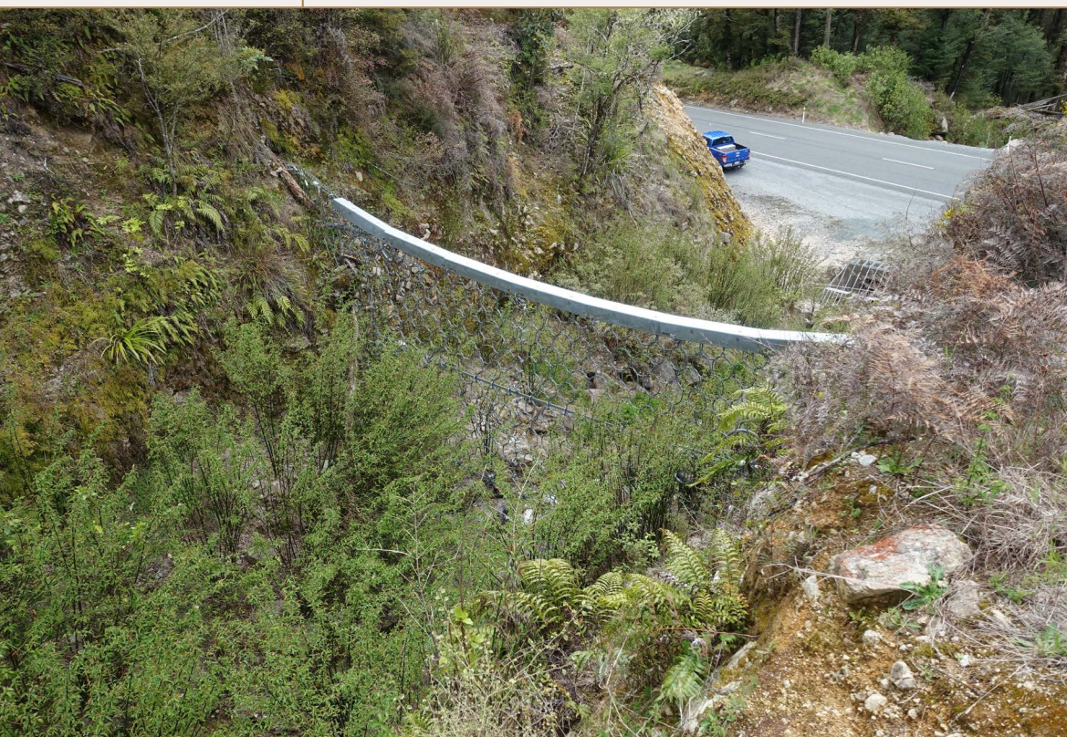
Figure 4. Springs Junction (South Island) – Shallow landslide barrier
