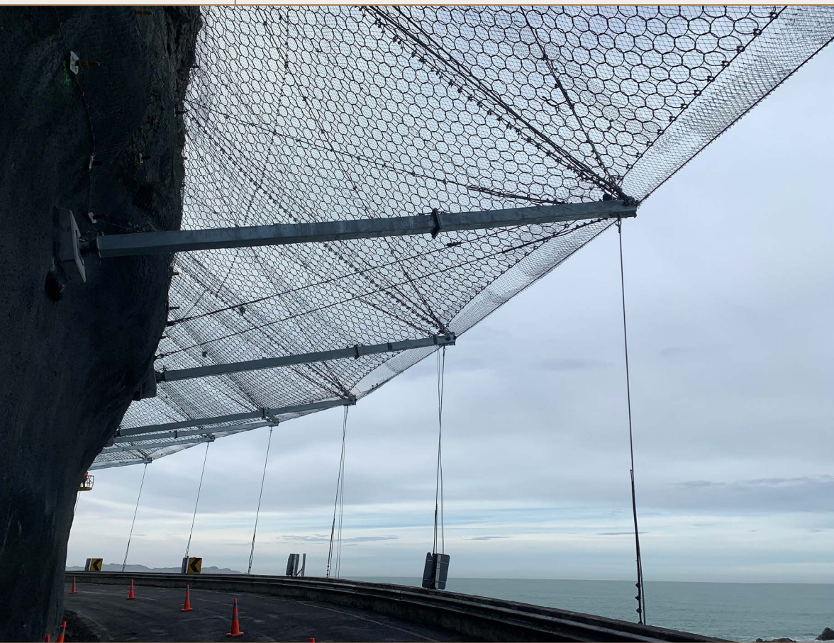
Figure 6. Kaikoura debris nets, installed to protect State Highway 1 and the adjacent railway line after the 2016 Kaikoura earthquake
